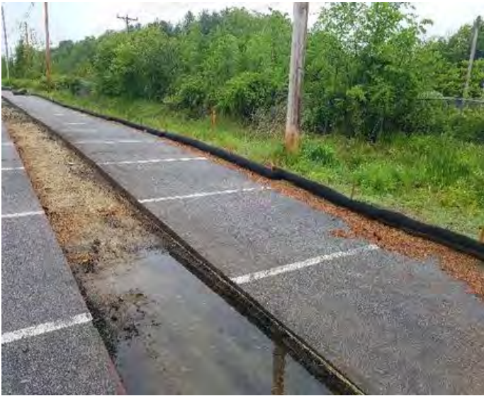
Fig 1: McCourt installed straw sock along trenching in A lot. Viewing northeast.
