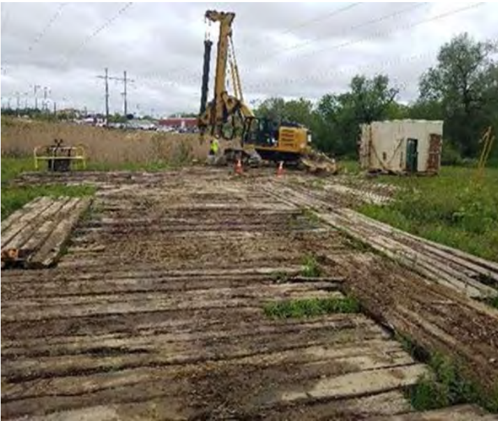
Fig 5: Timber matting implemented around Strs. F107-138,139. Viewing west.
