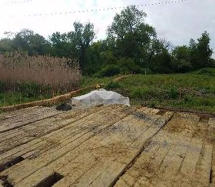
Fig 9: Poured foundation for Str. F107-138. Viewing northwest.
