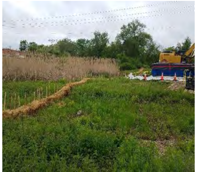
Fig 6: Straw bales installed between Str. F107-138 and wetland NW37. Viewing north.
