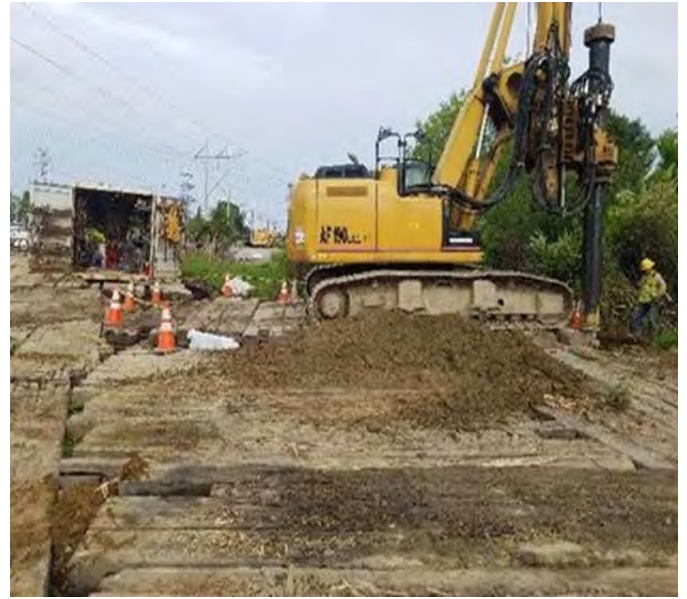
Fig 10: MJ drilling foundation location for Str. F107-139. Viewing east.
